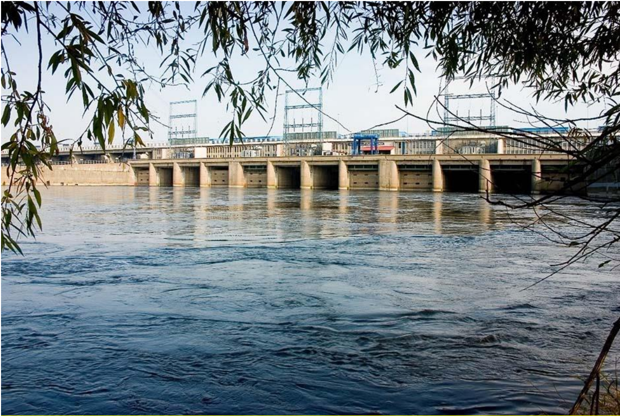
Włocławek Hydroelectric Power Station
