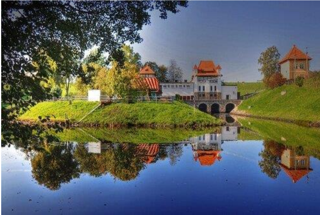
Straszyn hydro plant
