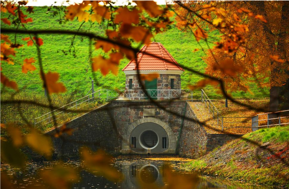
Straszyn hydro plant
