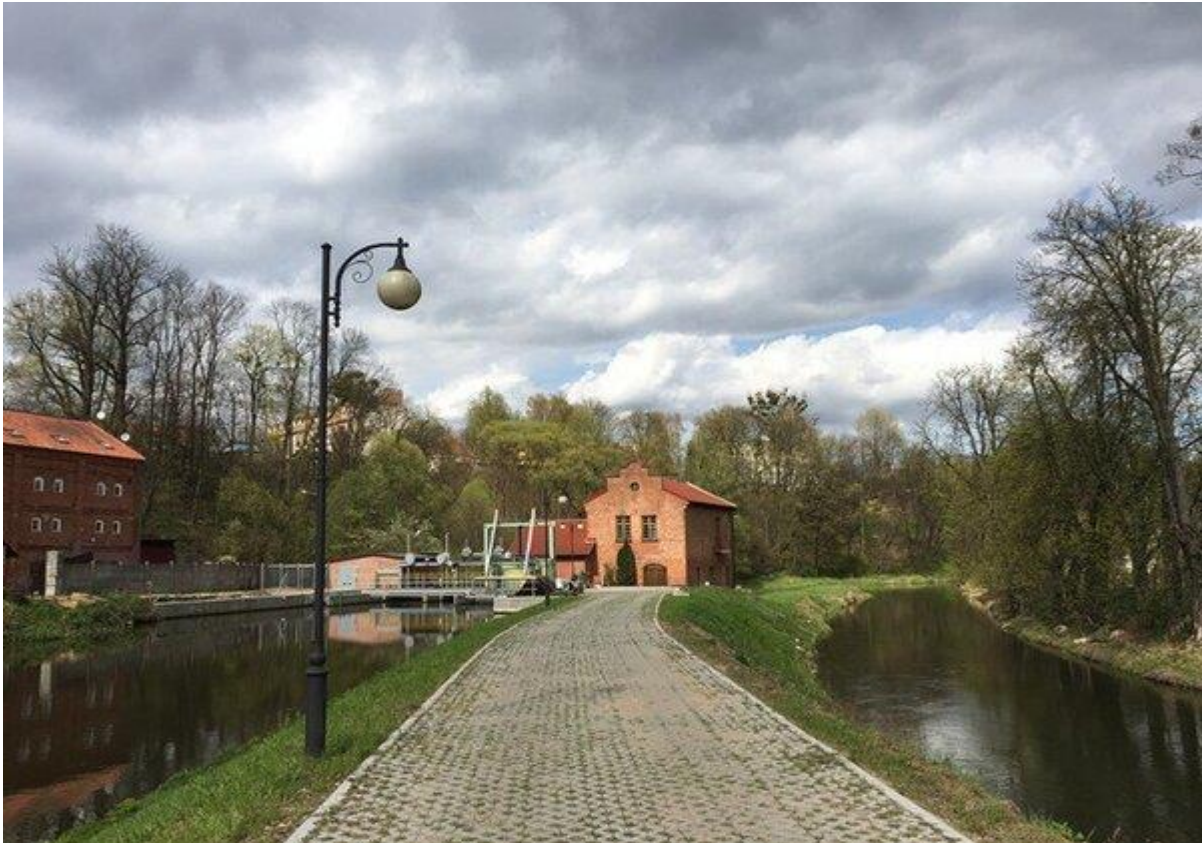
Lidzbark Hydro plant
